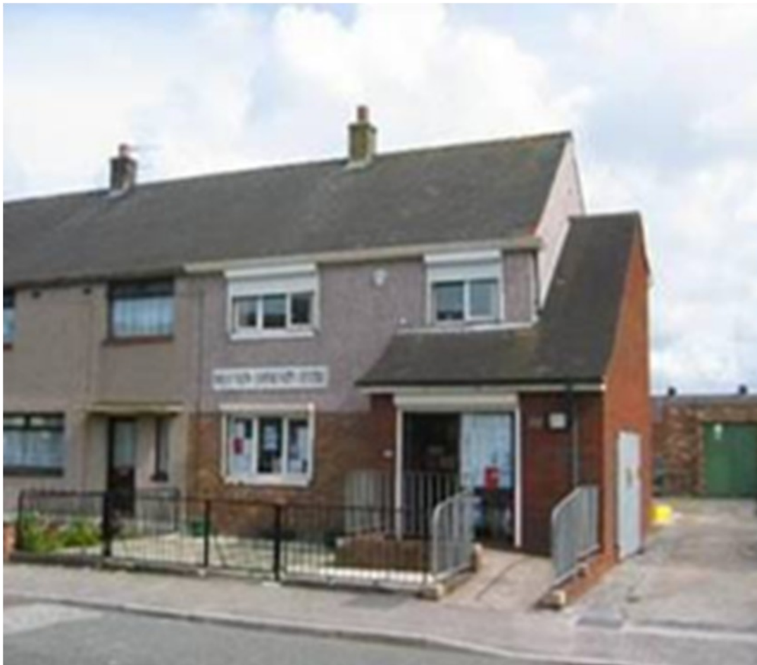
West View Community Centre, Eden Avenue
